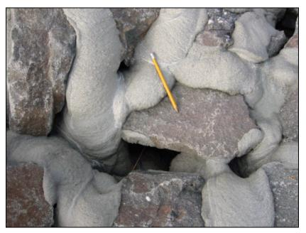
Figure 12.1. Close-up view of partially grouted riprap.
