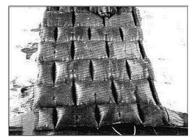
Figure 9.8. Articulating block mat appearance after filling (ODOT).
