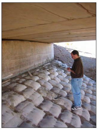
Figure 9.2. Grout-filled mat used for scour protection at a bridge abutment.
