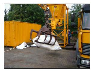
Figure 11.20. Handling a one-tonne sand-filled geotextile container. (photo from NCHRP Project 24-07(2), courtesy Colcrete – Von Essen Inc.)
