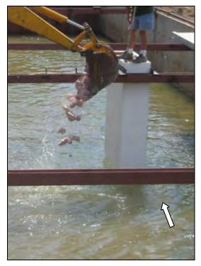
Figure 11.13. Installation of riprap around pier.
