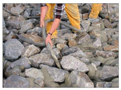
Figure 12.20. Grout placement by hand.
