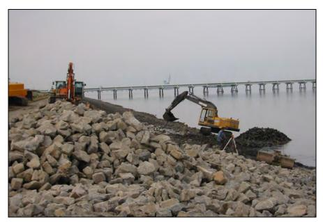
Figure 4.11. Placing riprap with hydraulic excavators.
