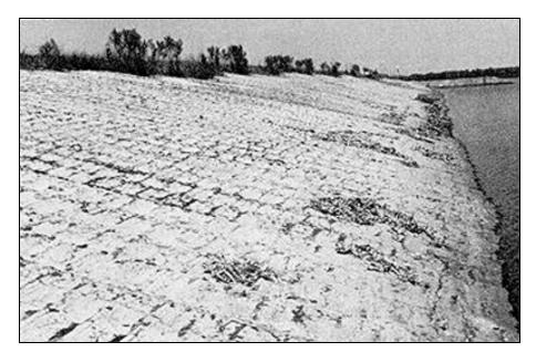
Figure 7.3. Soil cement placed in the plating method parallel to the slope (PCA).
