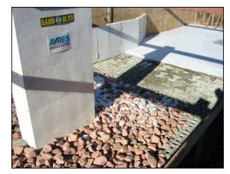
Figure 12.12. Loose riprap, ACB, and contraction wall installation (note loose riprap on the near side of the pier and partially grouted riprap on the far side).
