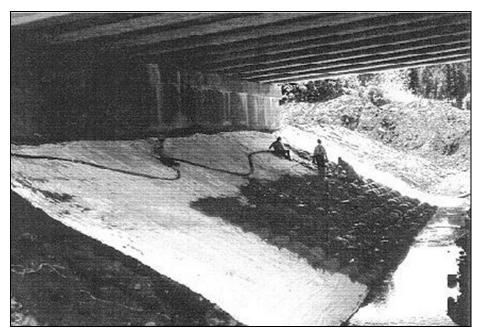
Figure 9.9. Installation of articulating grout filled mat proceeding upslope (ODOT).
