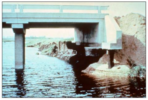
Figure 14.1. Scour of bridge abutment and approach embankment.
