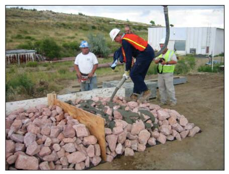
Figure 12.8. Preliminary trial grout application in the dry.
