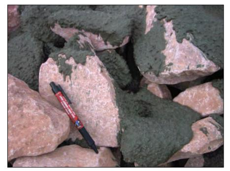
Figure 12.9. Surface of the riprap after partial grouting.
