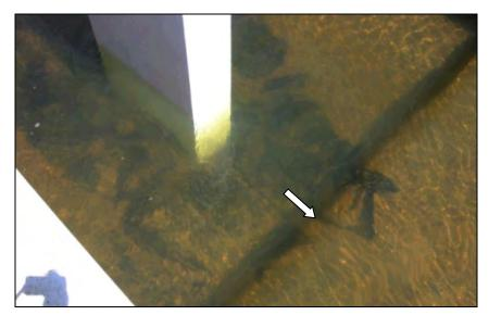
Figure 11.12. Geotextile containers after installation.
