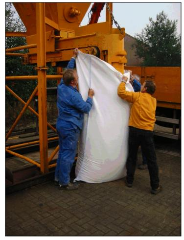
Figure 11.19. Filling geotextile container with sand. (photo from NCHRP Project 24-07(2), courtesy Colcrete – Von Essen Inc.
