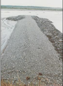
Figure 2.13. Impermeable spur field in top photograph with close-up shot of one spur in the lower photograph, vicinity of the Richardson Highway, Delta River, Alaska.
