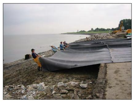
Figure 12.17. Hand placing geotextile prior to placing partially grouted riprap. Note sewn seam.
