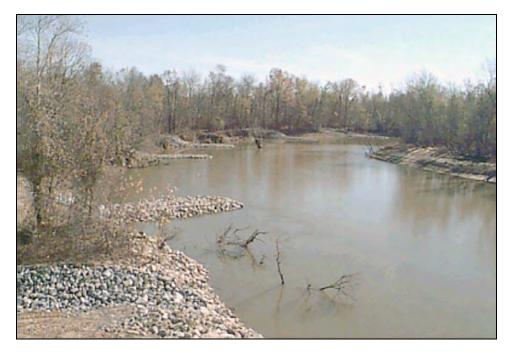
Figure 1.9. Bendway weirs on northbank of Hatchie River looking upstream (TDOT).
