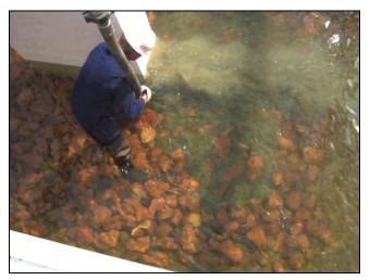
Figure 12.11. Underwater partial grouting of riprap.
