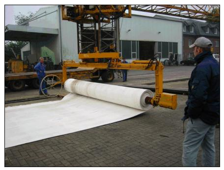
Figure 11.18. SandMat<sup>™</sup> geocomposite blanket being unrolled. (photo from NCHRP Project 24-07(2), courtesy Colcrete – Von Essen Inc.)
