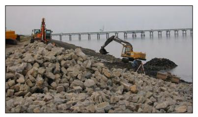
Figure 12.18. Placing riprap with hydraulic excavators.
