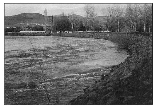
Figure 1.7. Submerged bendway weirs on the Yakima River, Washington at high flow (WSDOT).
