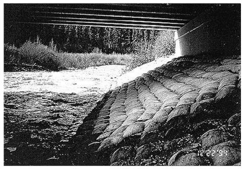
Figure 9.10. ABM underneath Salmon Creek Bridge (ODOT).
