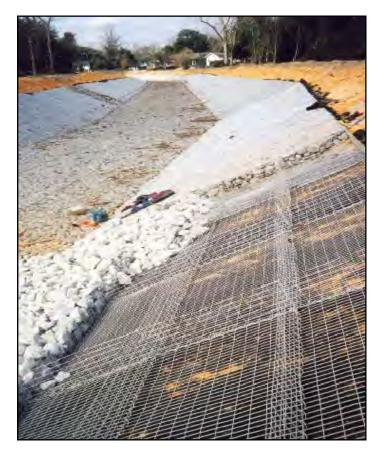
Figure 10.2. Field installation of gabion mattresses on channel bed and banks.
